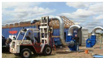
Boilermaker's Lodge with Shipping Containers/Roof Structure and Installation of Ductwork, Modular Two-Piece Booths, and Exhaust Fans
