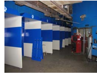
Cleveland Community College Oskar Air Welding Booth Installation
