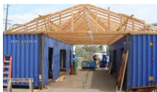
Boilermaker's Lodge with Shipping Containers/Roof Structure and Installation of Ductwork, Modular Two-Piece Booths, and Exhaust Fans
